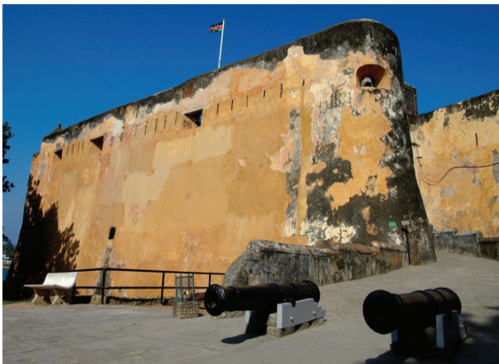
Plate 116: Fort Jesus World Heritage Site/ Photo courtesy of NMK
