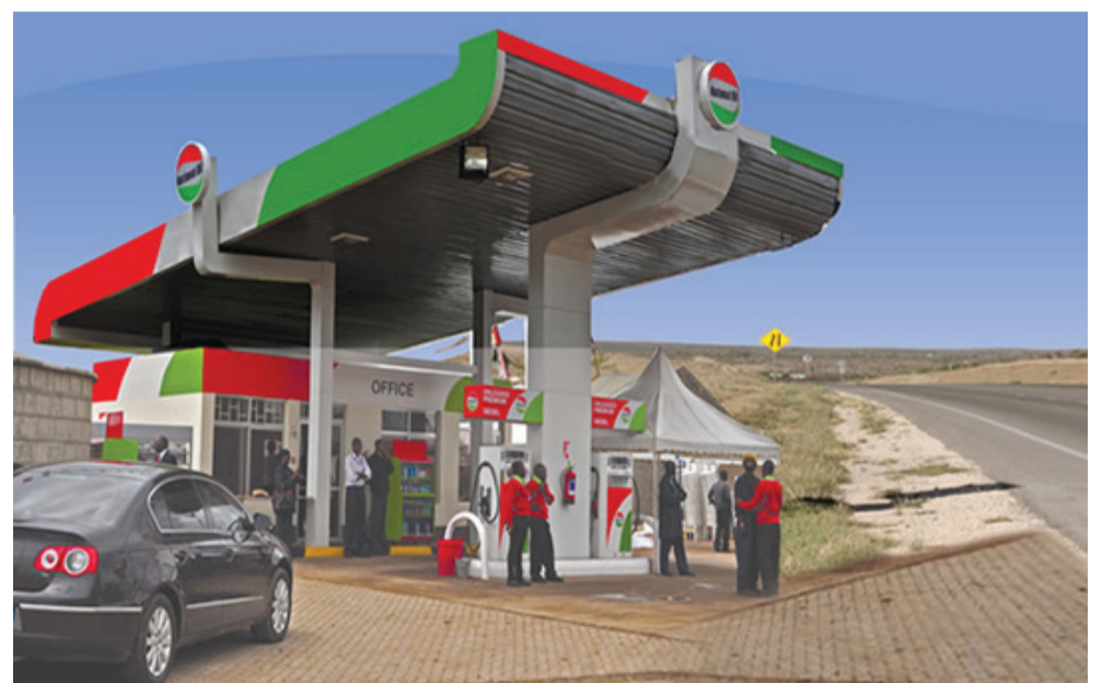
Plate 92: Downstream petroleum distribution to end users, MoEP
